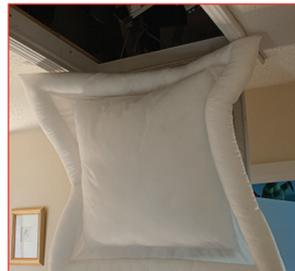
4. Close hatch ensuring the flap makes a seal between the hatch and its housing.
